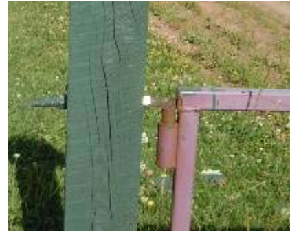
Threaded bolt extending past wood gatepost
