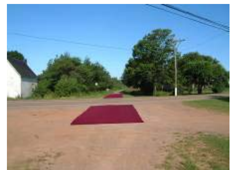
“Welcome Mat” Surface treatment at intersections
