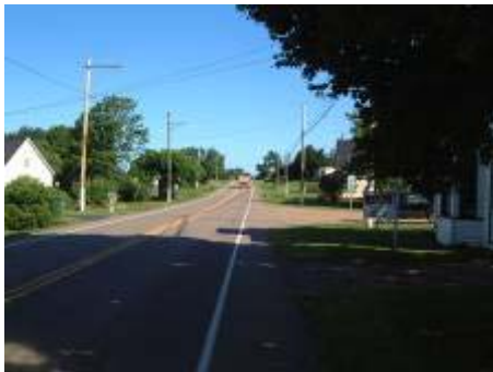
Trail crossing and signs are not visible
