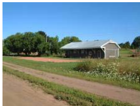
Old Railway Station at York
